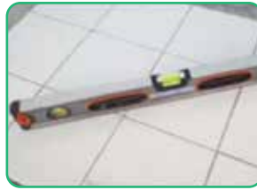
5. Cek Kerataan Pasangan Keramik Ceramic Flatness Checking
