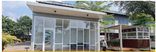
Mandalika Circuit, Lombok - Building Progress
