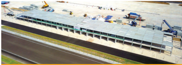
Mandalika Circuit, Lombok - Building Progress
